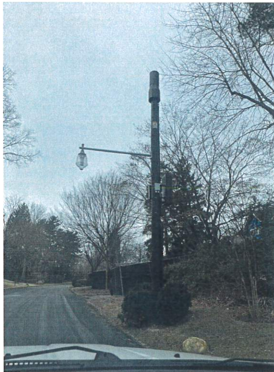
Figure 17 – Typical DAS Node Installation
