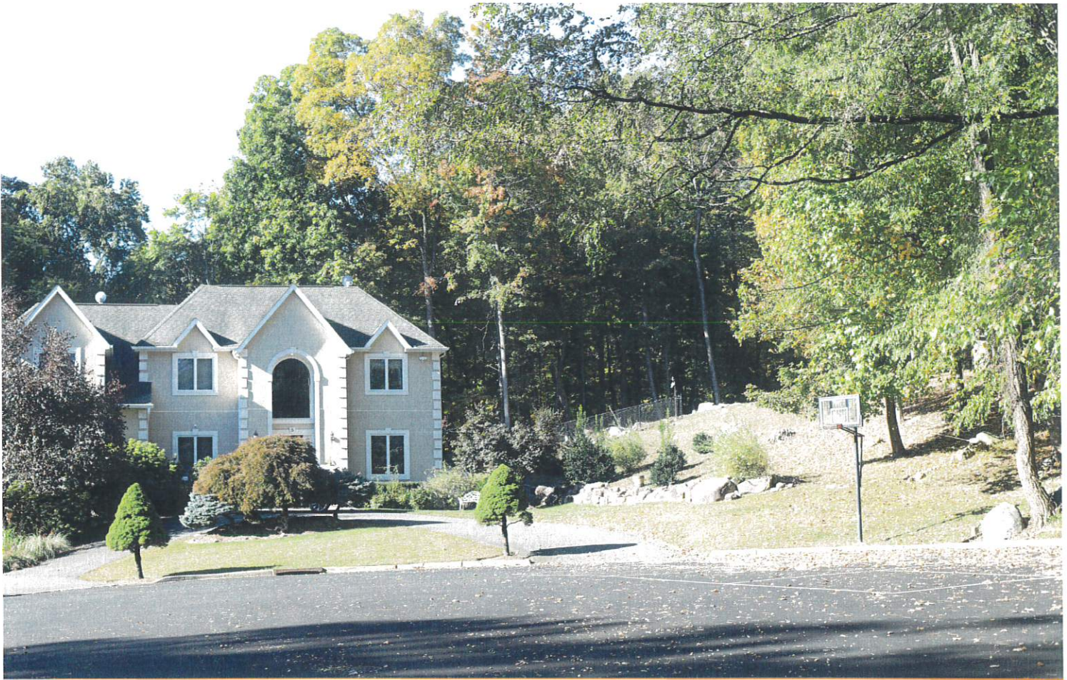
Photo 11 - Regis Ct. cul-de-sac EXISTING CONDITION
