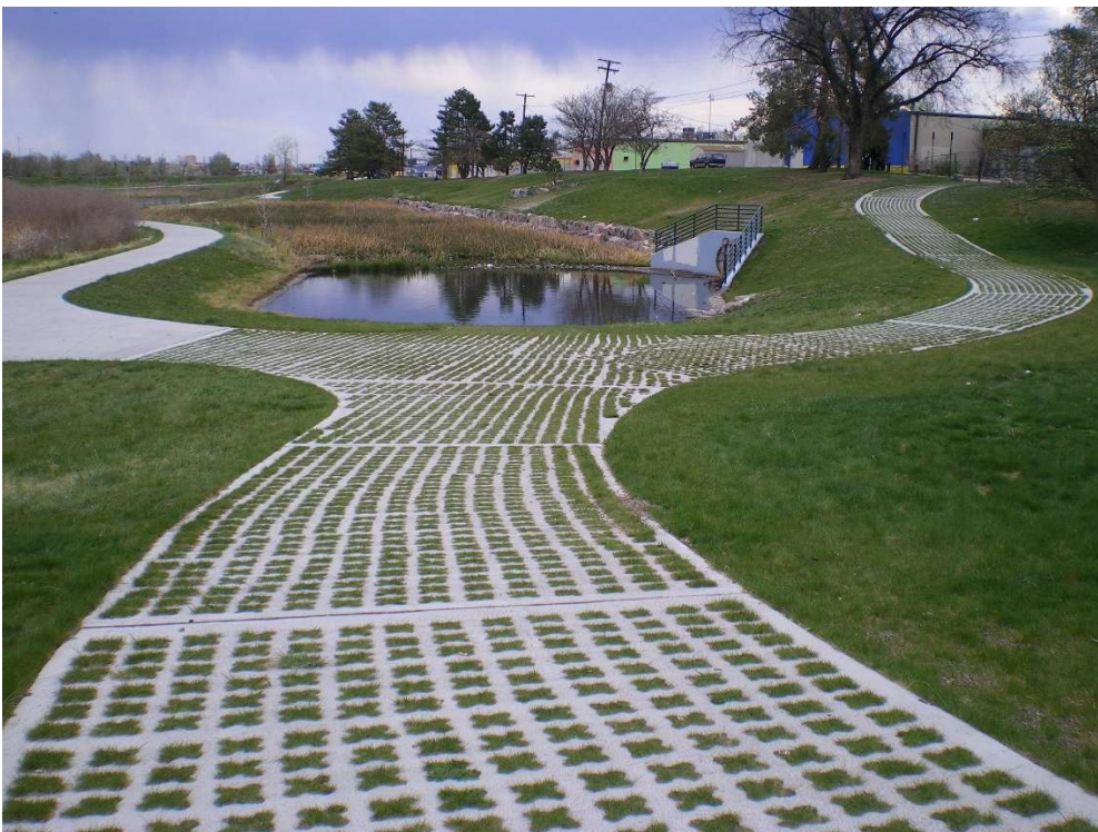
Photo 2: Grasscrete 1 year after installation
