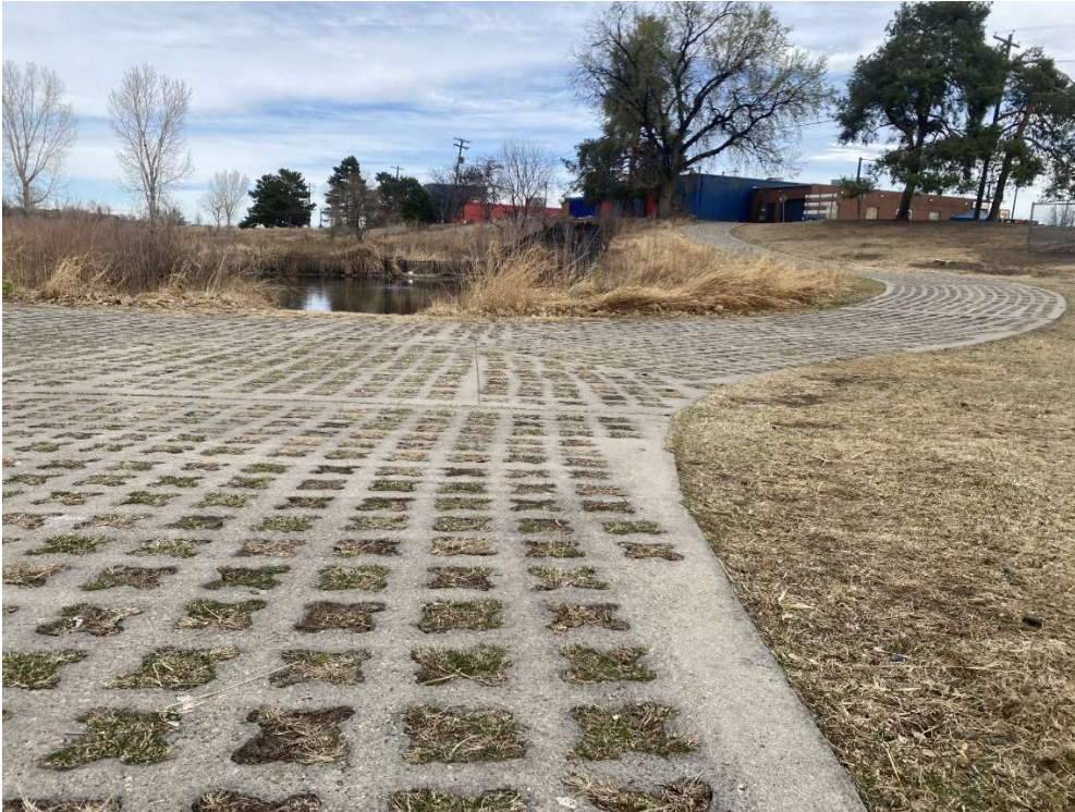
Photo 1: Grasscrete immediately after installation
